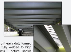
Structure consists of heavy duty formed steel side girders fully welded to high strength steel joists. (Picture shows under side of ramp)
