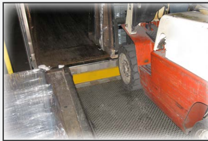
The barrier is designed to allow for end-loading at the loading dock.
