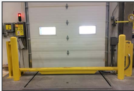
Collision protection for the overhead door.
