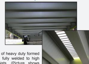
Structure consists of heavy duty formed steel side girders fully welded to high strength steel joists. (Picture shows under side of ramp)
